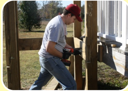
HEATH WORKING ON THE WHEELCHAIR RAMP
