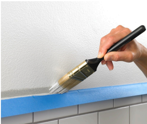
Use paint brush on area next to painters' tape
